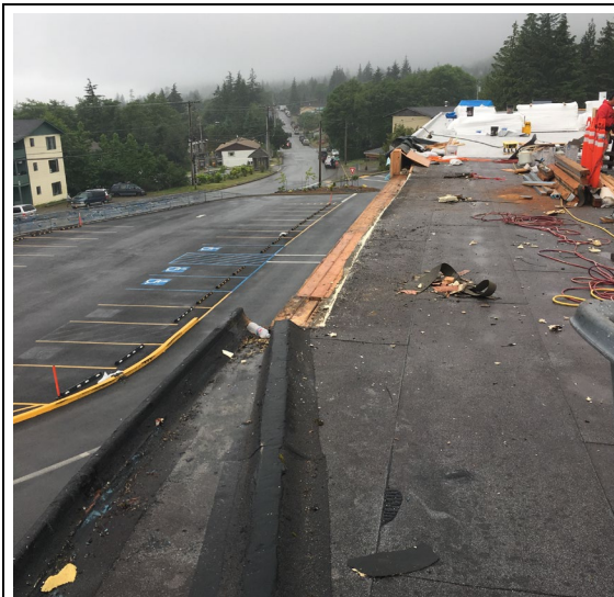
Photo #7 – South section of parapet (In front of fan room)
