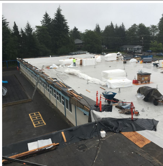
Photo #2 – East side of the main roof (taken from gym roof)
