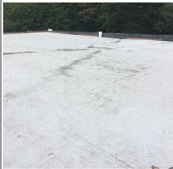
Photo #9 – East roof (facing northeast)
