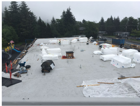
Photo #1 – East side of the main roof (taken from gym roof)
