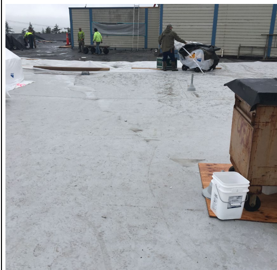
Photo #8 – East roof (facing west towards gym)
