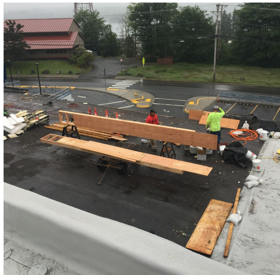
Photo #6 – South section of parapet (In front of fan room)
