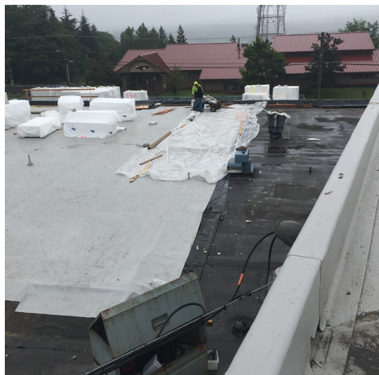
Photo #3 – East main roof looking south along grid #11.
